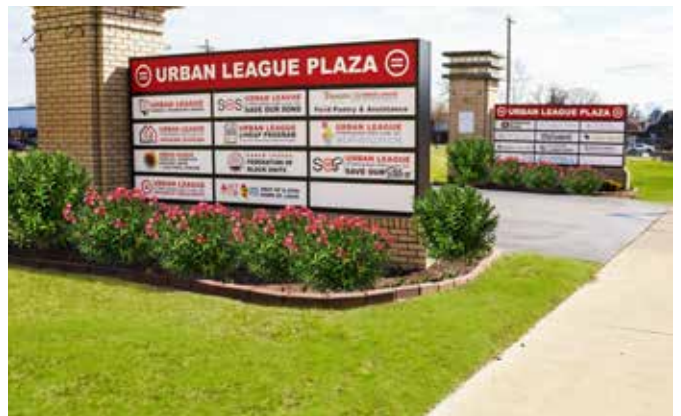
New Lighting & Signage
